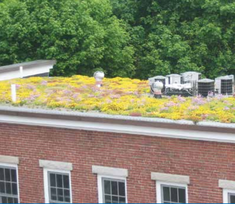
Above: The green roof at Whipple Annex in Ipswich, MA helps protect the adjacent Ipswich River from pollution and erosion
