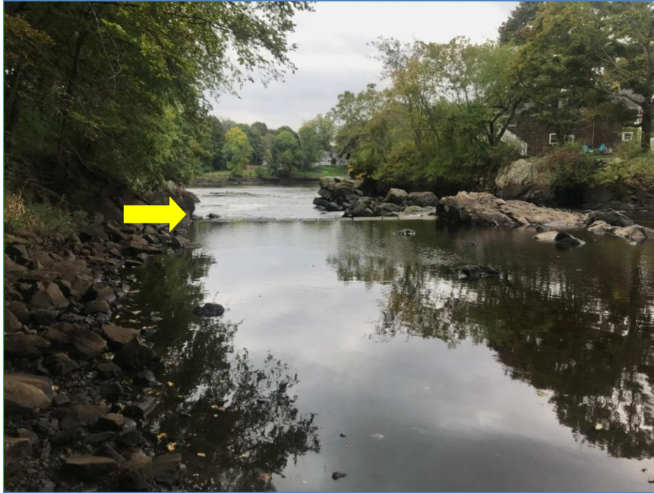
Photo 3. View of left bank of Ipswich River (looking downstream). A portion of an old dam restricts water flow during low tide cycles. The dam, coupled with a rocky outcrop located in the center of the river creates a different flow regime on the left and right banks of the river at this location.
