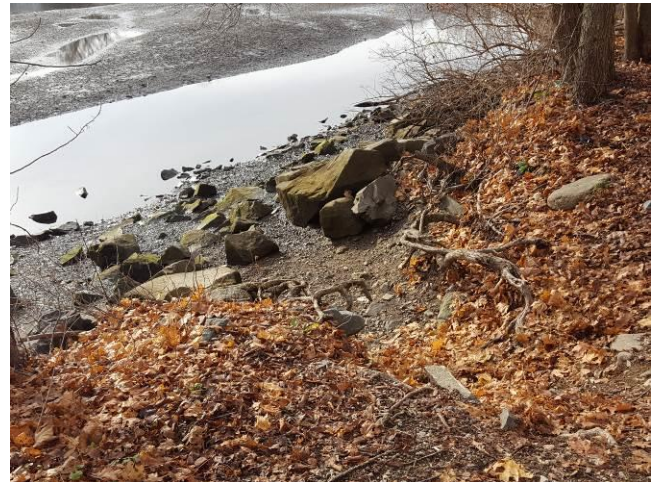
Image 2#: Area 2 – Section of Bank Erosion
