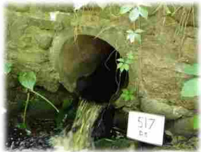
Figure 48. Outlet of road-stream at Winthrop Street (Site #517). This perched crossing was the highest priority crossing identified by screening tools in the Town of Hamilton.
