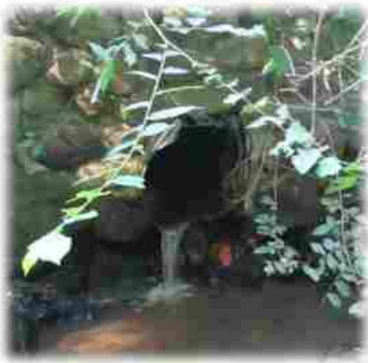
Figure 13. Perched outlet of non-tidal crossing at Coleman Road in Newbury (Site #1054)
